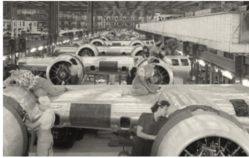
Vega Plant 1, B-17 wing subassembly line, 1942.
