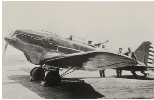
The XP-900/YP-24 was the first Lockheed fighter, first U.S. military monoplane fighter and first U.S. military aircraft with fully retractable landing gear, 1931.
