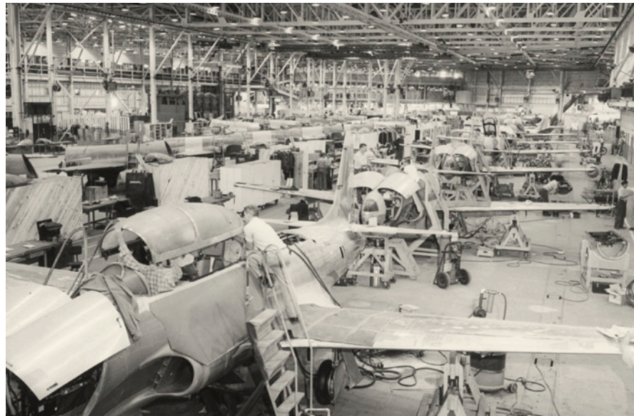
Production line at Skunk Works for the TF-80 operational trainer, 1948.
