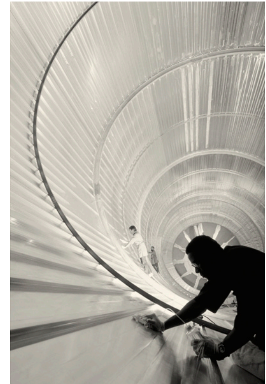
A 28-foot-diameter liquid-oxygen tank, an interior structure of the space shuttle's giant external tank, is cleaned with solvent following pressurization tests, 1984.
