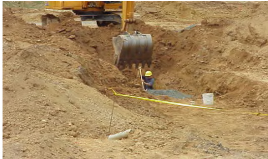
Not properly sloped, benched, etc.
